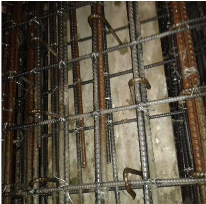
Photo: columns during retrofitting phases
