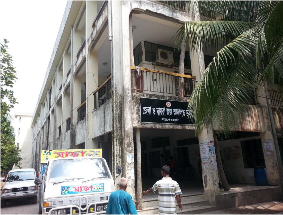
Fig: Bagherhat Judge court Building
