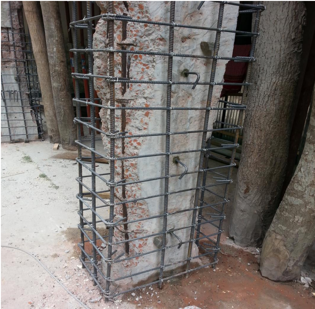
Photo: Column During retrofitting
