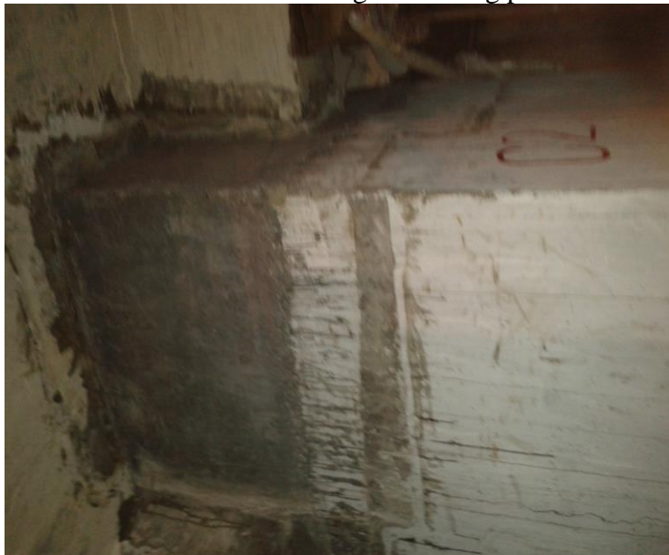
Photo: Column after retrofitting
